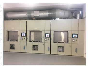
The decision was taken to line the new cremators with refractory bricks which are more durable than conventional linings, they retain more heat in the brickwork resulting in less gas usage, and the cremators are fitted with smart software that monitors the conditions in the cremators and maintains the required temperature to meet operating conditions.
